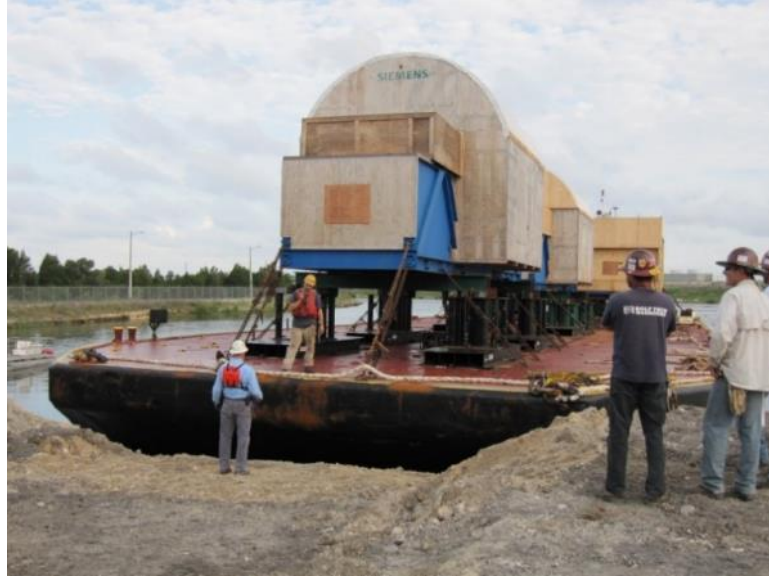
Turbine Component Unloading at Crystal River
