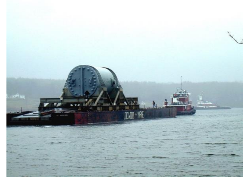
Reactor Pressure Vessel Shipping at Maine Yankee
