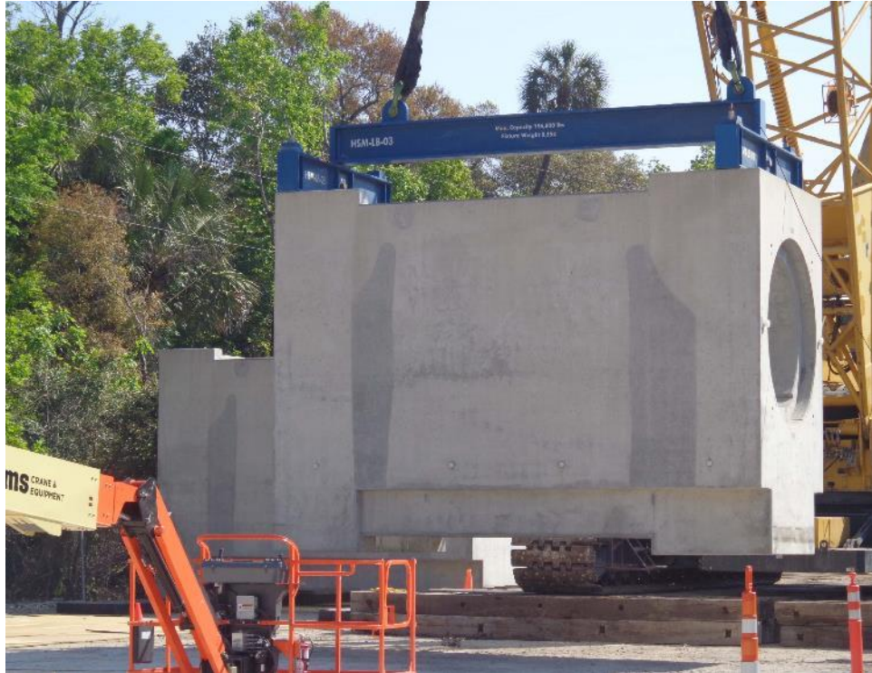
Horizontal Storage Module Being Unloaded from Railcar
