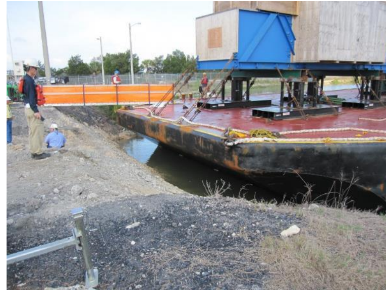
Docking Barge with Turbine Components
