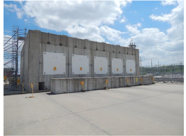
Horizontal Storage Modules at Fort Calhoun (Fort Calhoun, Nebraska)
