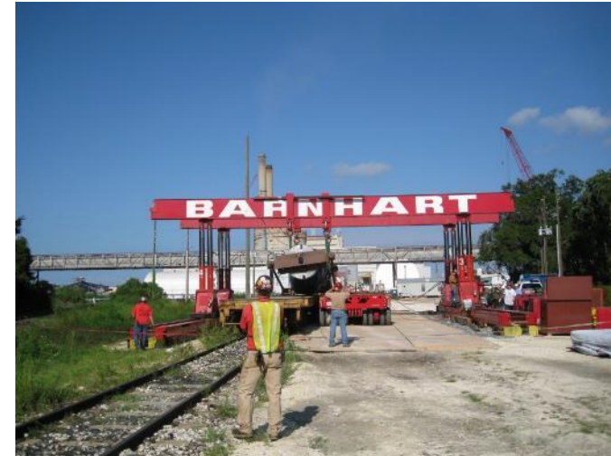
Unloading Generator Rotor
