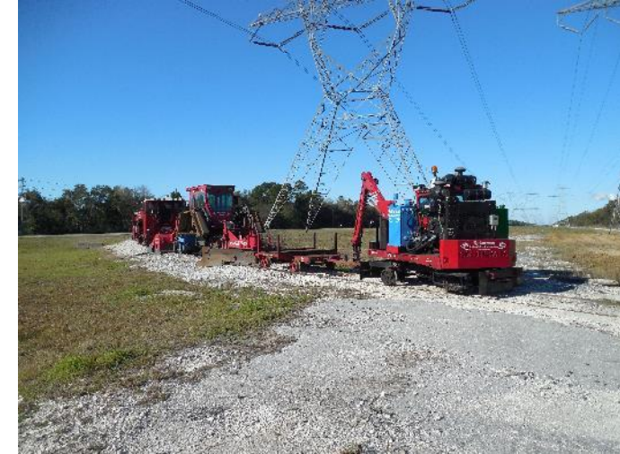
Track Maintenance Equipment Staged at Mine Spur
