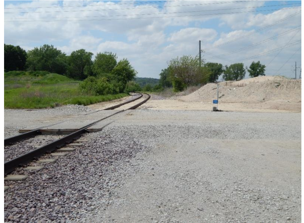
Rail Spur Looking Northwest
