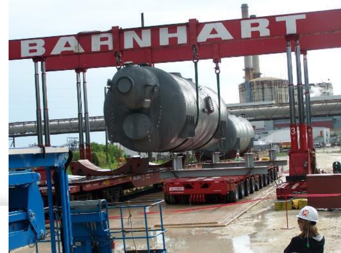
Unloading New MSRs
