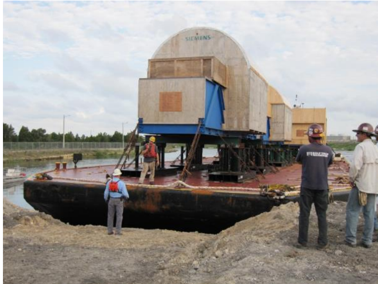
Barge with Turbine Components Approaching Ramp
