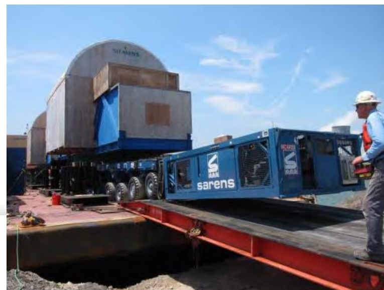
Turbine Components Being Unloaded Using Self-Propelled Modular Transporter (SPMT)
