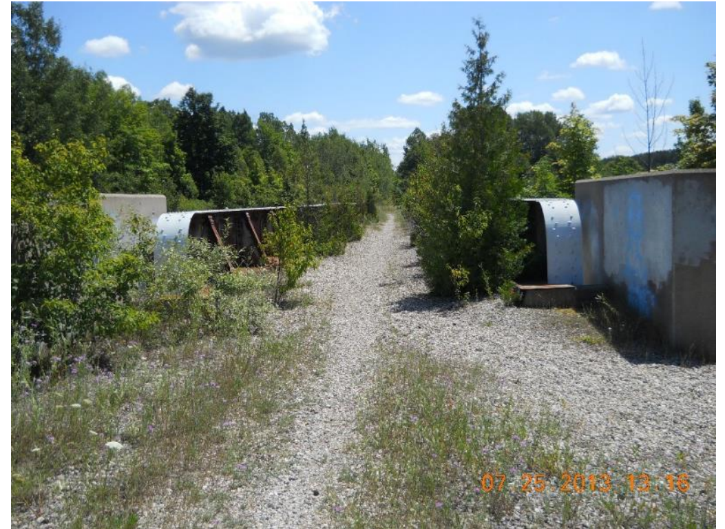
Top of Low Overhead Bridge
