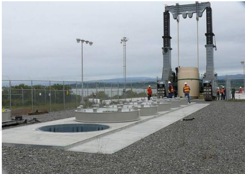
Underground Storage Modules at Humboldt Bay (Eureka, California)
