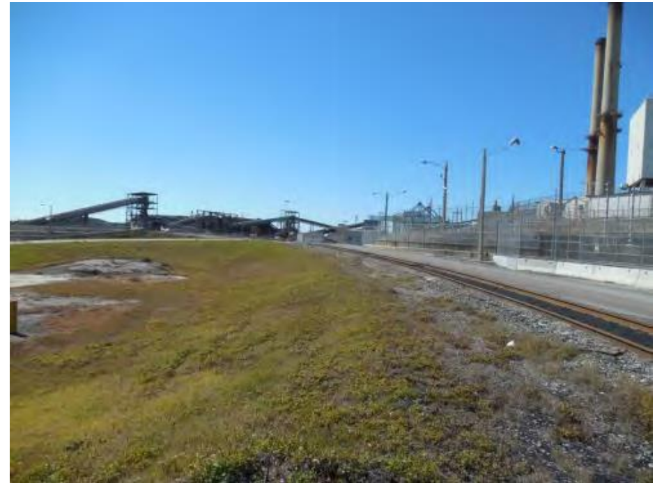
Onsite Rail Facing West
