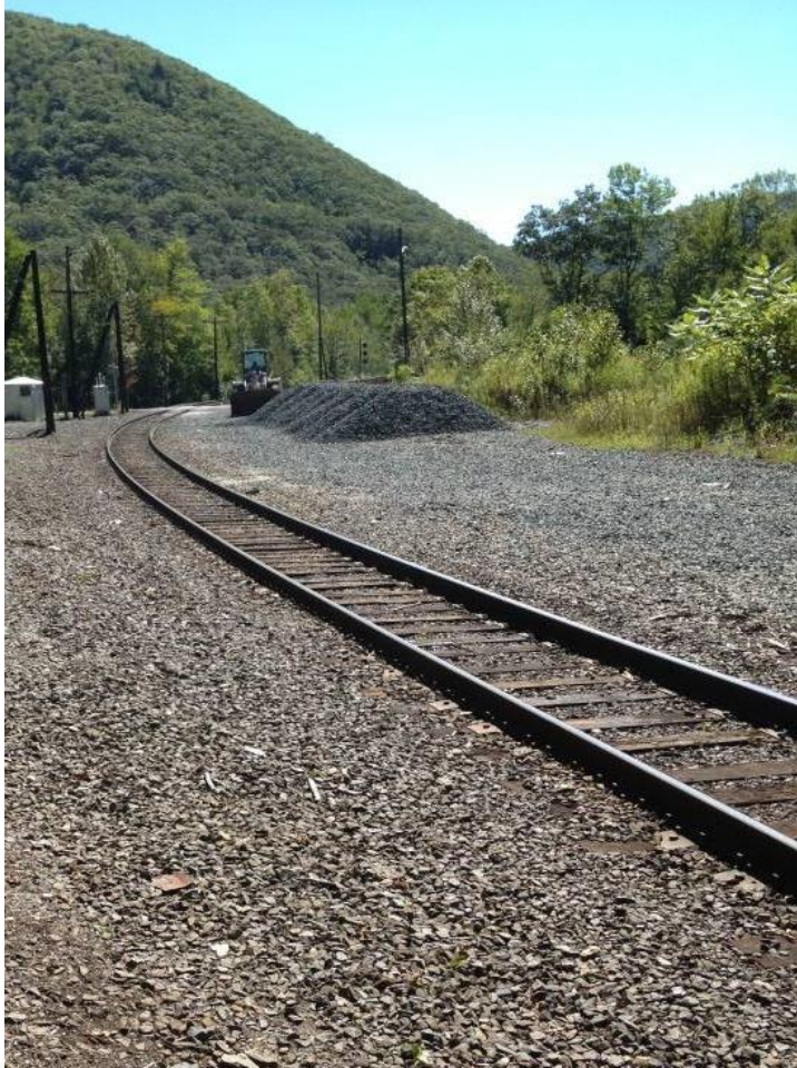
Offsite Rail Access at Hoosac Tunnel
