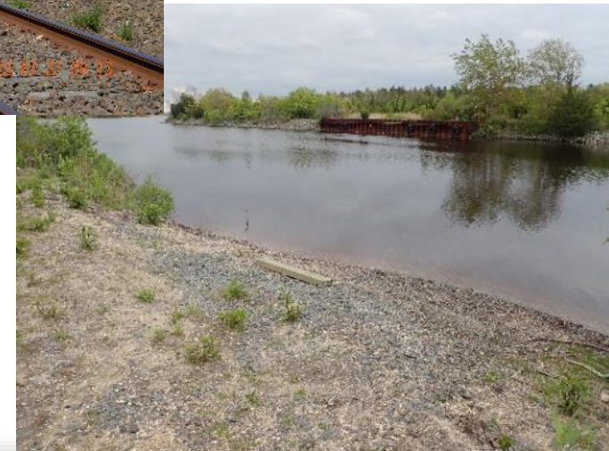
Oyster Creek Barge Landing Access Road
