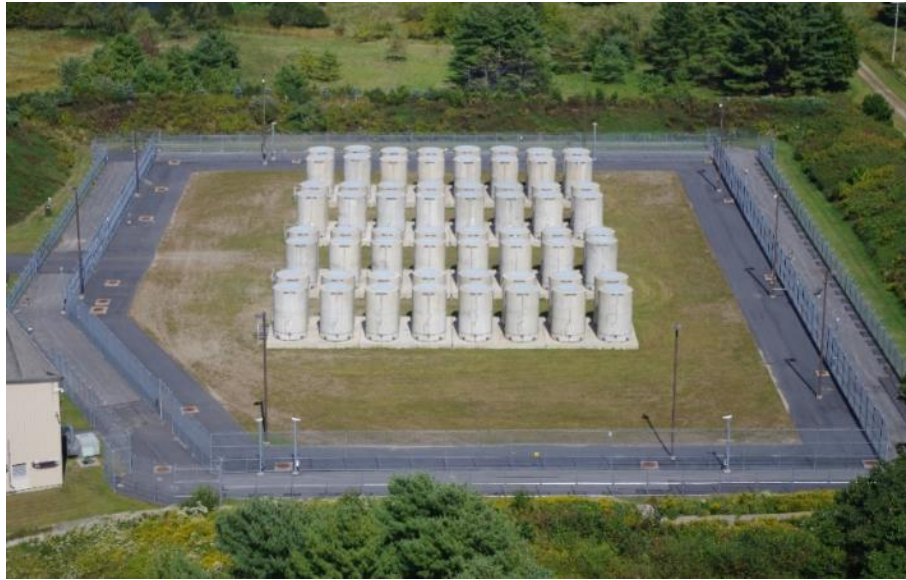
Vertical Concrete Casks at Maine Yankee (Wiscasset, Maine)
