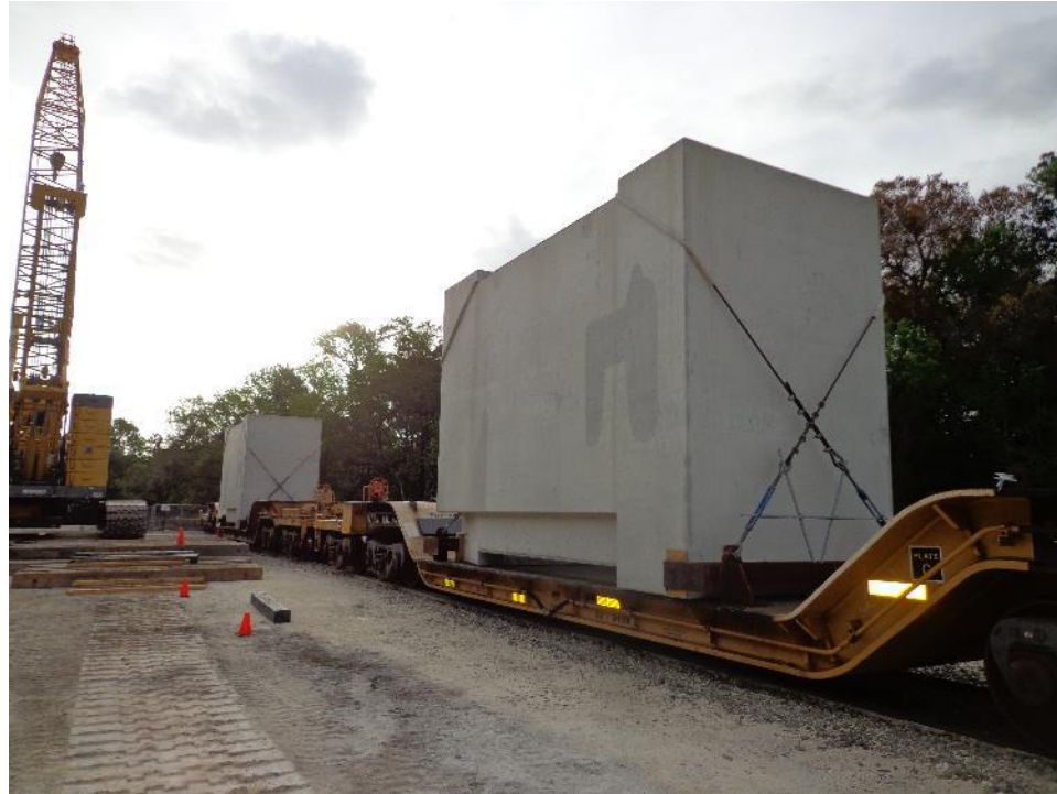
Received 12 horizontal storage modules Each horizontal storage module weighed 189,000 lb.
