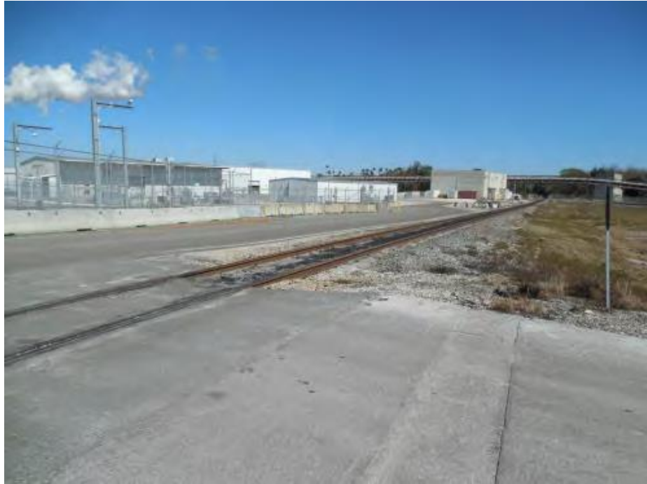
Onsite Rail Facing East
