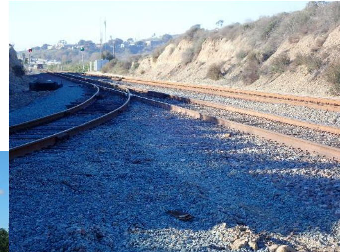
Junction of Onsite Rail Spur with BNSF Mainline at San Onofre
