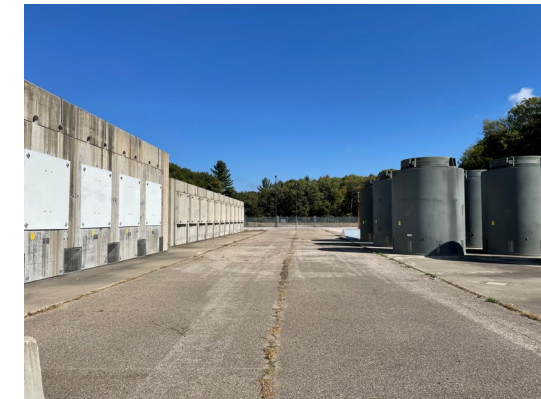
Palisades ISFSI, October 2022
