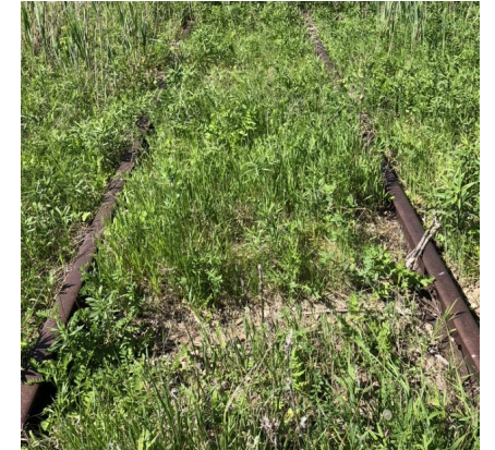
Rail spur condition near GE Hitachi Morris Site, May 2022
