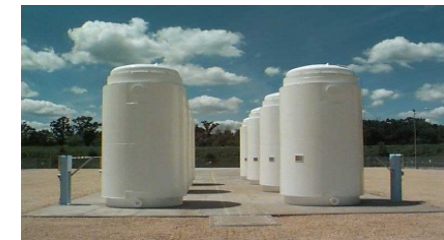
PR Fuel in Storage Casks
