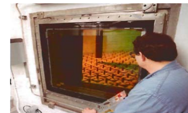
RR Fuel Dry Storage Facility
