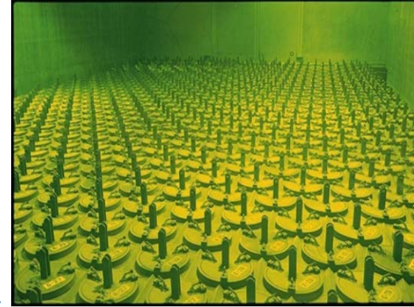
INL CPP-603 dry storage facility
