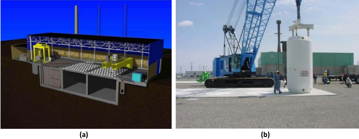
Figure 4. Hanford Spent Nuclear Fuel Storage Facilities. (a) Canister Storage Building; (b) Interim Storage Cask Being Placed on a Concrete Pad at the 200 Area Interim Storage Area (McCormack 2014b).
