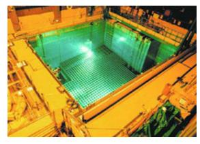
Figure 1. Example of a Spent Fuel Pool at a Reactor. Source: NRC (2021b)
